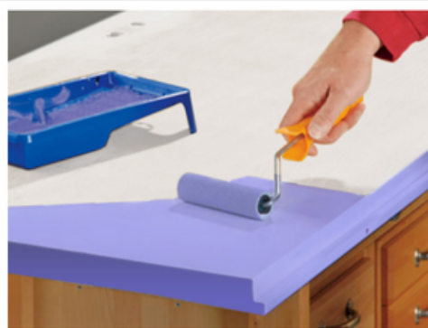
Next, a finish coat is applied on both sides.
